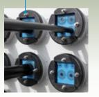
Base station shelter: Round sealing solution for openings in port hole plates.
