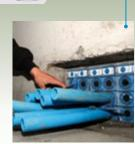
**FTTH:** Conduits for fiber optics sealed in the foundation of network shelter.
